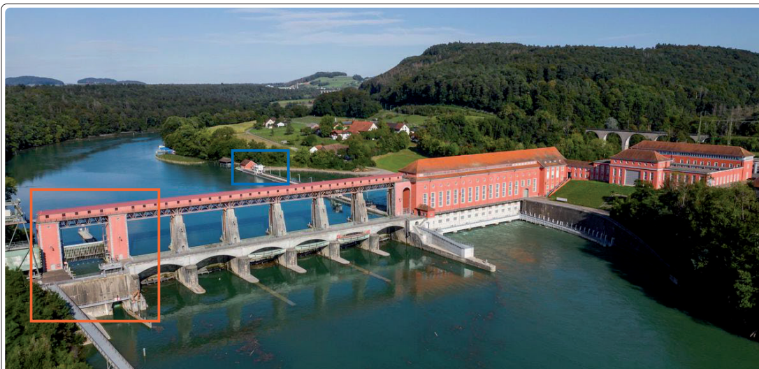
Fig. 3: The hydropower plant in Eglisau: The water lock (orange) and the water filter (blue) in the inlet basin
